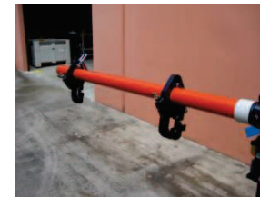
Figure 24 - Fixed Bracket in Position
