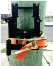
Figure 9 - Attaching Bracket to Pole
